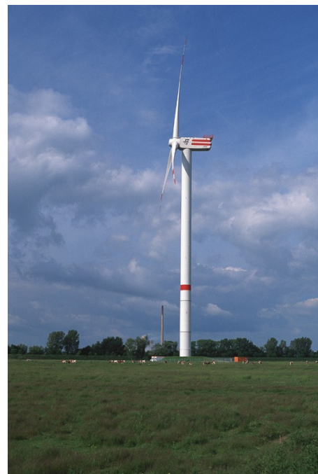
21. irudia. REpower 5M. Alemanian, 2005 (Itur.: REpower Systems-en kortesia, copyright REpower Systems).
